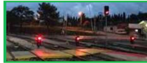
(signals and level crossing at the background – ÇAMLIK)
